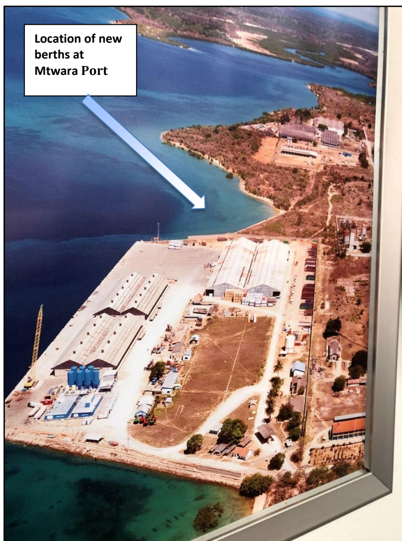
Figure 2: Aerial view of Mtwara Port
